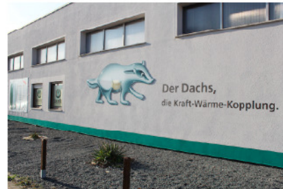
▶ SenerTec Center in Darmstadt
